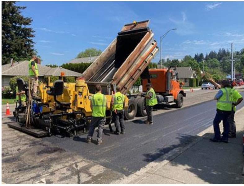
Road construction project at Hardie Avenue SW.
